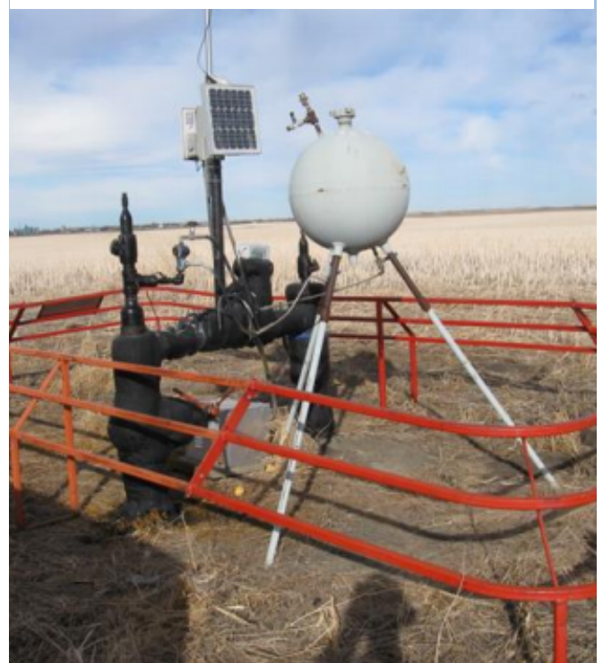
Figure 5: Methanol sphere installation
