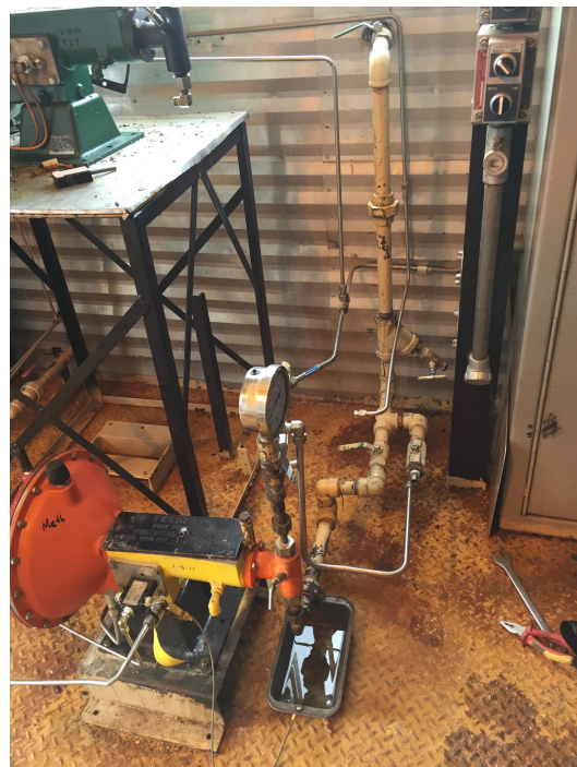
Figure 1: Gas-driven methanol diaphragm pump
